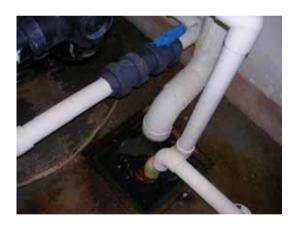
Pic2 4" drain pipe from the elevated water storage tanks appears in the center of this picture taken at the water discharge pit.
