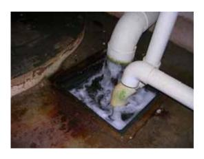
Pic3 Discharge of overflowed water. Now the tanks at the top of the pump house become full.
