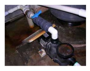
Pic6 Do not remove the plastic cover to protect the pump from drips of seawater.
